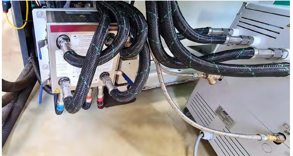
On the left side: the Water Switch Box; on the right: the rear of a temperature controller. This installation arrangement makes it possible to keep the hose connections short. On both sides of the Water Switch Box, the manual levers for the ball valves are visible.
